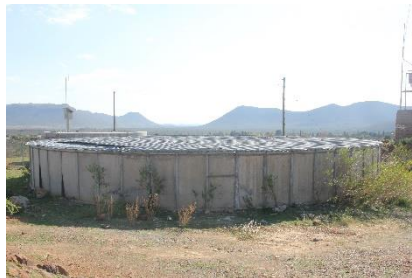
Murraysburg 0.500 MI. Fence was vandalized and removed. Galvanised roof sheets were stolen
