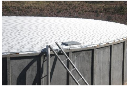
Merweville 0.200 MI Reservoir (Cover not locked)
