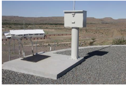
Merweville 0.400 MI Reservoir (Cover not locked)
