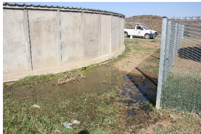
Murraysburg 0.500 MI reservoir (Leaking)
